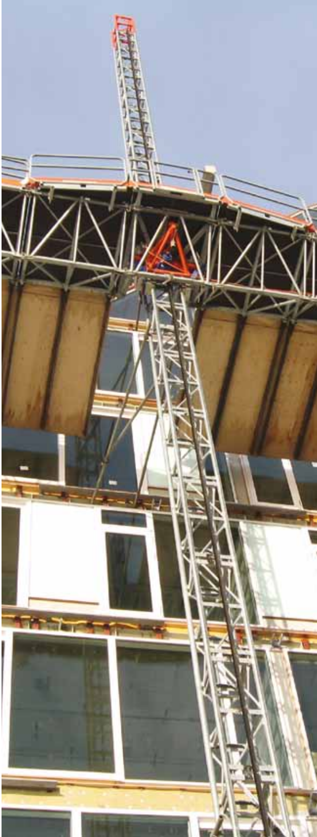
The main selling point of MCWPs is that they are a quicker, more cost-effective alternative to scaffolding
