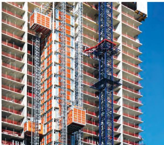
Specialist hoists in action during the construction of the 75-storey Landmark Pinnacle residential tower in Canary Wharf, east London
