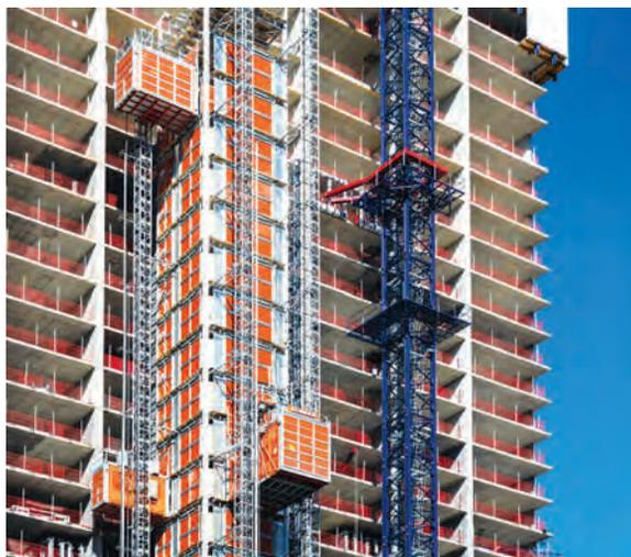
Specialist hoists in action during the construction of the 75-storey Landmark Pinnacle residential tower in Canary Wharf, east London
