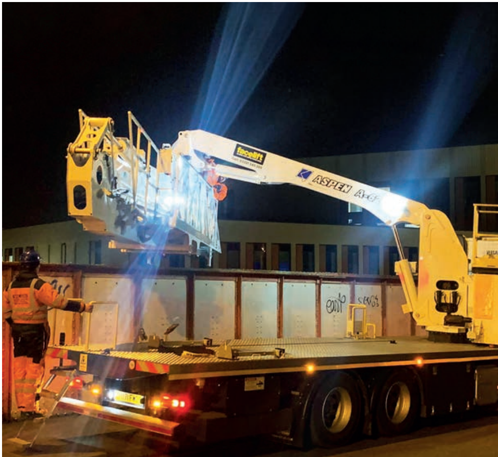
Facelift's new Aspen A-62 in action at Liverpool Lime Street station
